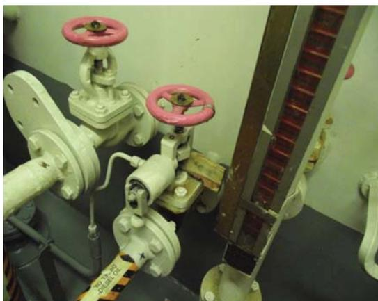
QCV blocked utilizing a wooden block to hold the valve in the open position.
