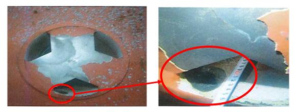
Picture 2 Corrosion on/around welded parts between distance pieces and bluff bodies
