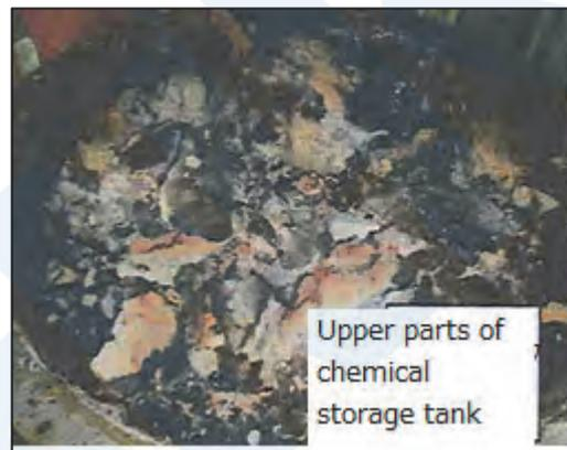
Photo 2 Upper part of burned-out chemicals storage tank
