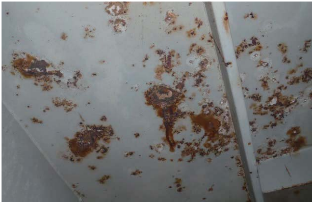
Corrosion holes of strength deck
