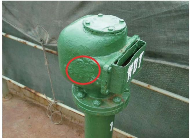
Inappropriate temporary repaired by putty
