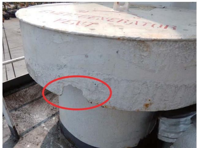
Wastage of the casing of ventilator
