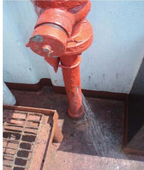
Leakage of fire line
