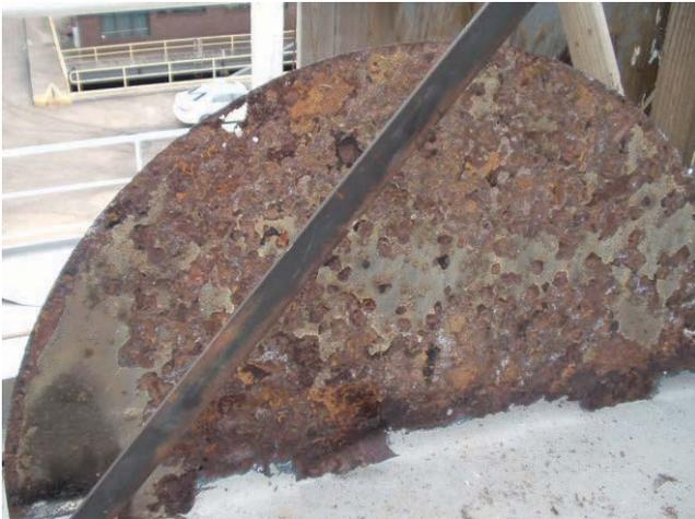
Wastage/Corrosion holes in fire damper flap
