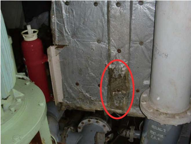
Partly missing A-60 class insulation
