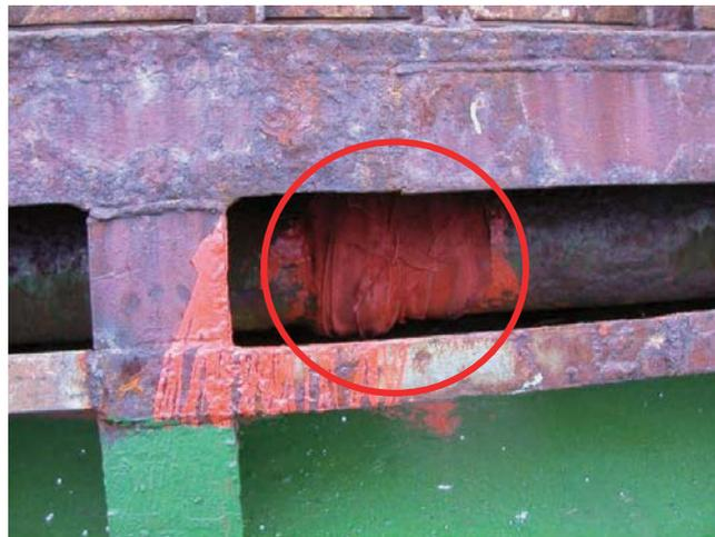
Inappropriate repair by cloth
