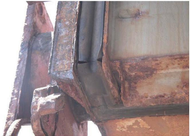
Deteriorated and cracked rubber packing
