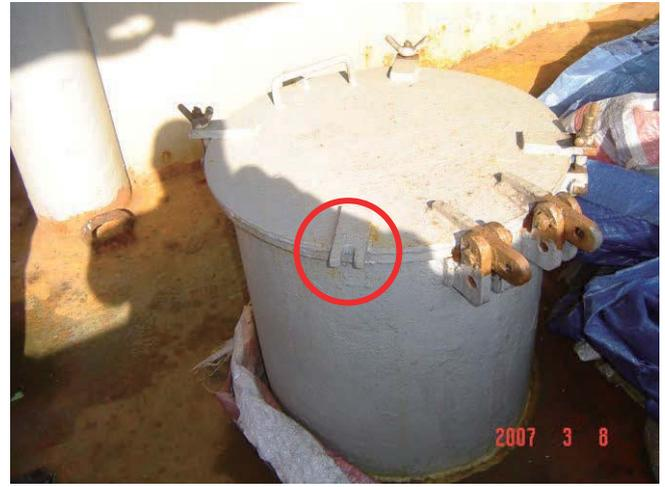
Missing nut and bracket with bolt
