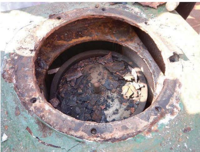
Excess Corrosion of inside of air pipe head
