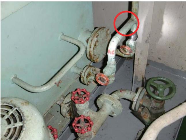
Inappropriate repairs by rubber patch and plastic putty
