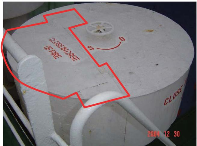
Inappropriate temporary repair by tape
