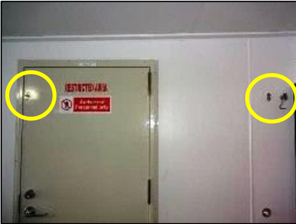
Hold-back hook fitted on self-closing door
