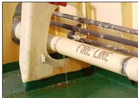
Leakage from fire main
