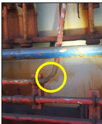
Corroded CO 2 lines
