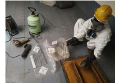
Packing of asbestos-containing material (ACM) in special bag
