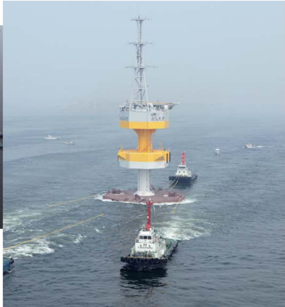
Transportation of floating sub-station
