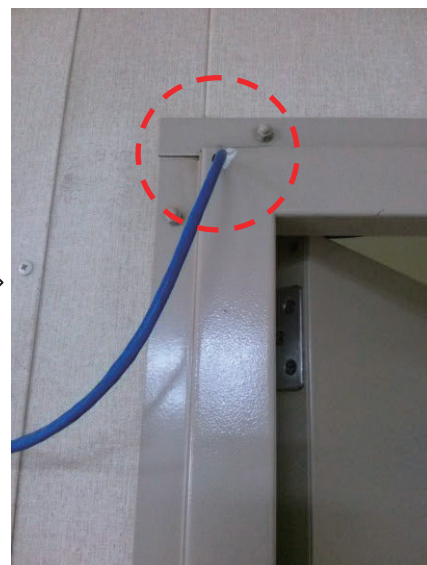
Improper cable penetration (through fire door frame)
