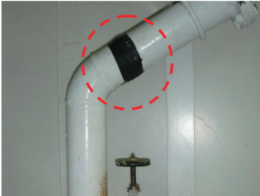
Oil leakage and accumulation
