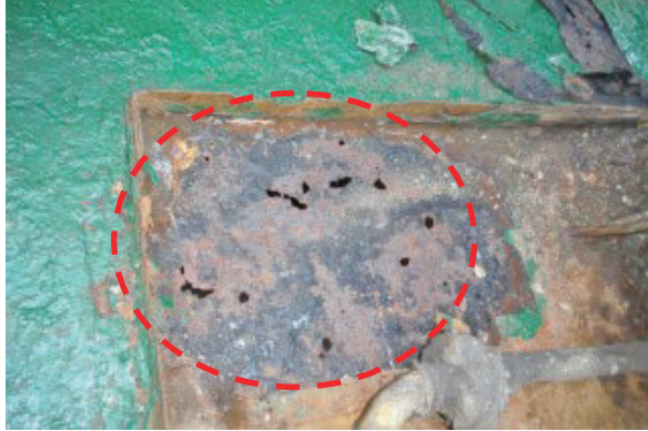
Corrosion holes on strength deck
