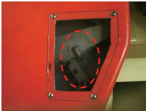
Improper reset of on load release gear interlock lever
