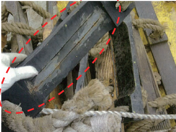
Poor condition of embarkation ladder
