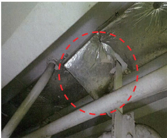
Detached insulation on underside of deck
