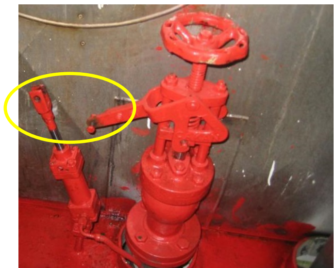
Disconnected control cylinder
