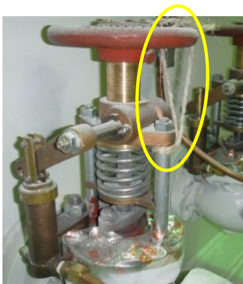
Quick closing valve lashed by rope
