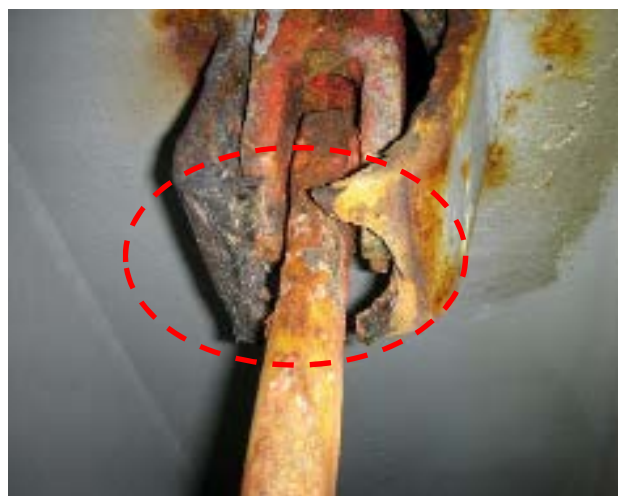
Wastage/damage of securing device crutch
