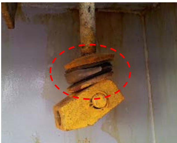
Damaged rubber washer
