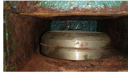
Missing/broken post
