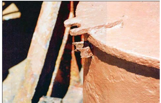
Hatchway securing device missing.
