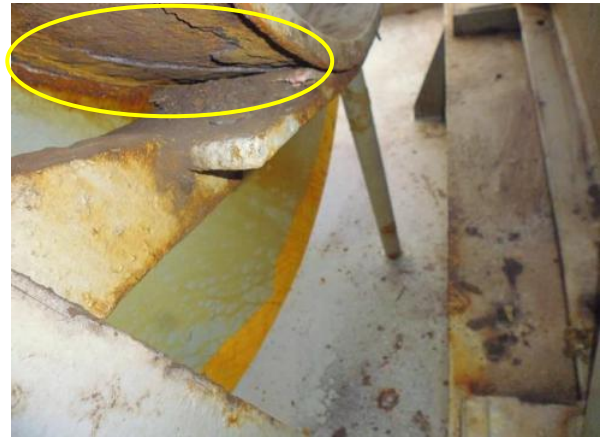
Poorly maintained windlass brake.
