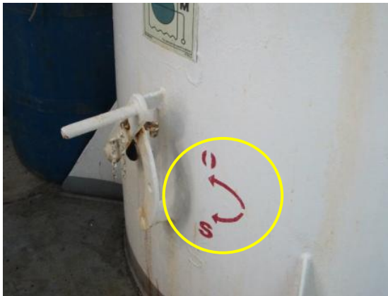
"Open-shut" positions clearly marked on ventilation trunk.
