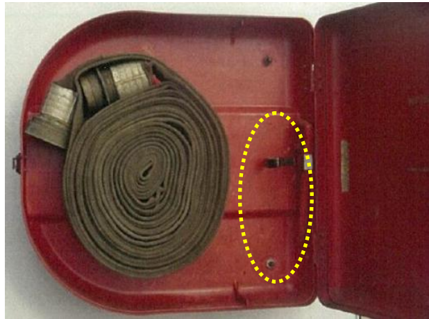
Hose nozzle missing.
