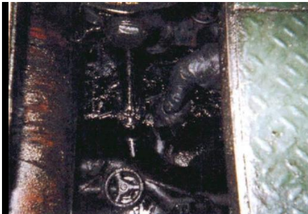
Tank top of engine room oily.
