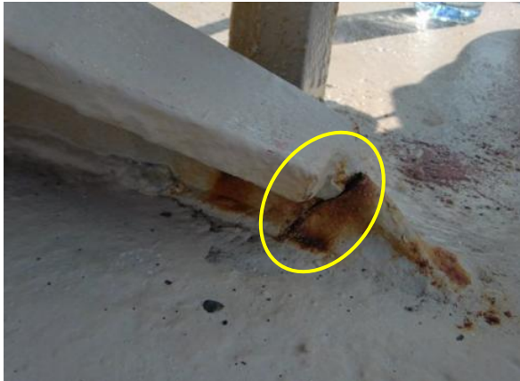
Cracked hatch coaming end bracket.
