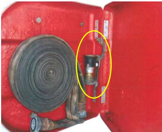
Properly fitted hose nozzle.
