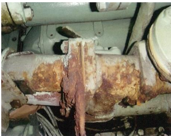
Badly corroded and leaking piping.
