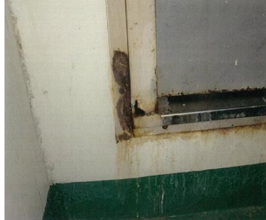
Worn-out and partially wasted fire door frame.
