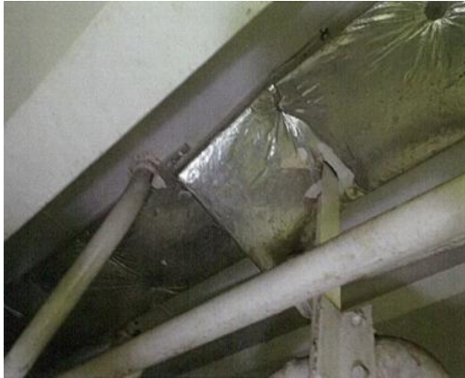
Deteriorated insulation on underside of deck.
