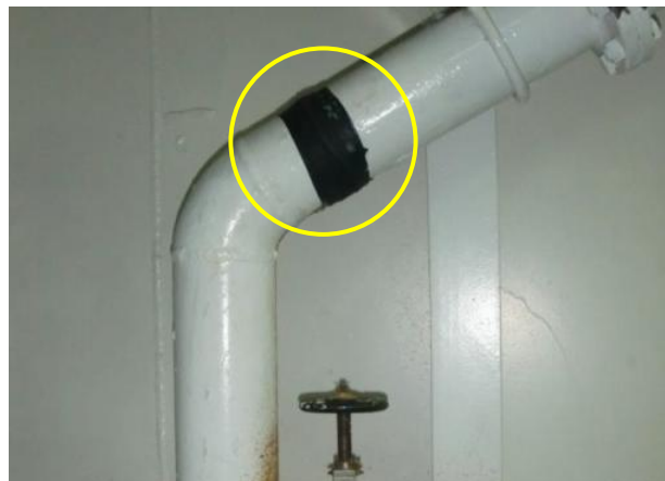
Pipe temporarily repaired with rubber patch.
