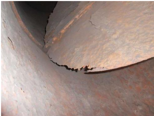
Fire damper flap wasted.
