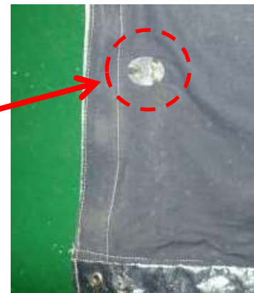
Interior (Metal exposed in side)
