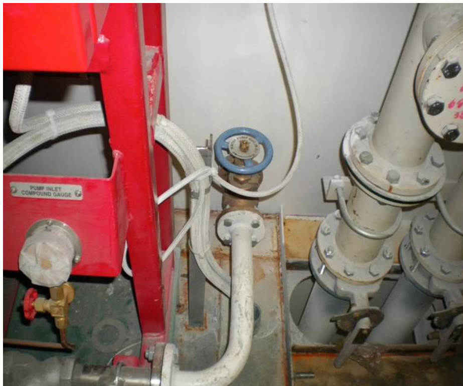
(1) Water supply valves to be always opened
