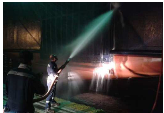
Hose test to confirm weather tightness
