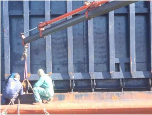
Condition and clearance of supporting hinges
