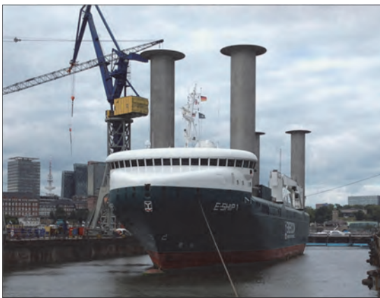
Figure 6 General view of the E-Ship 1 12)
