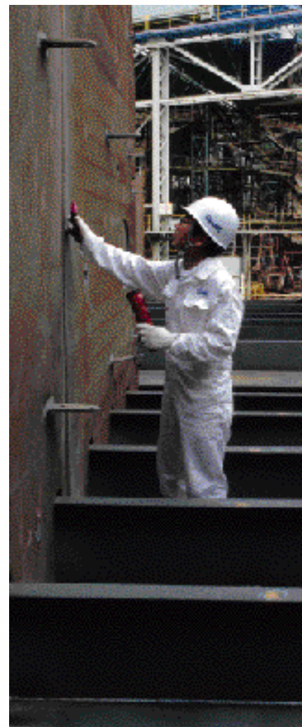
Re-checking of some welds
