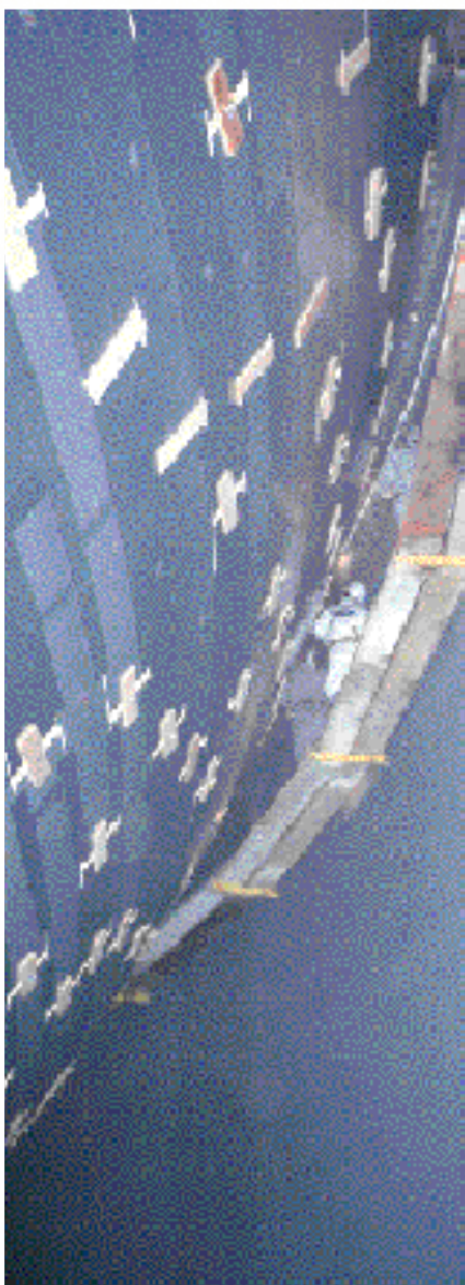
LNG Tank as seen from below
