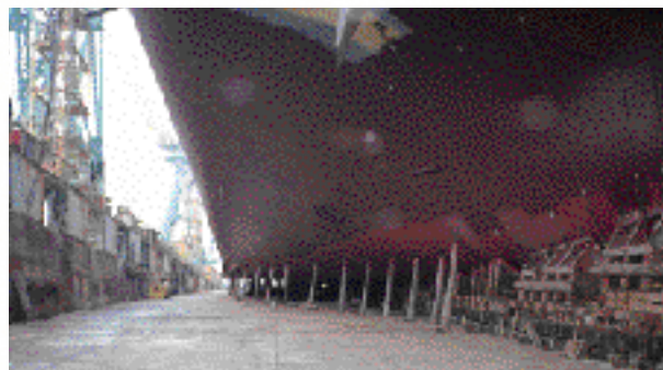
Slipway Launch Setup
