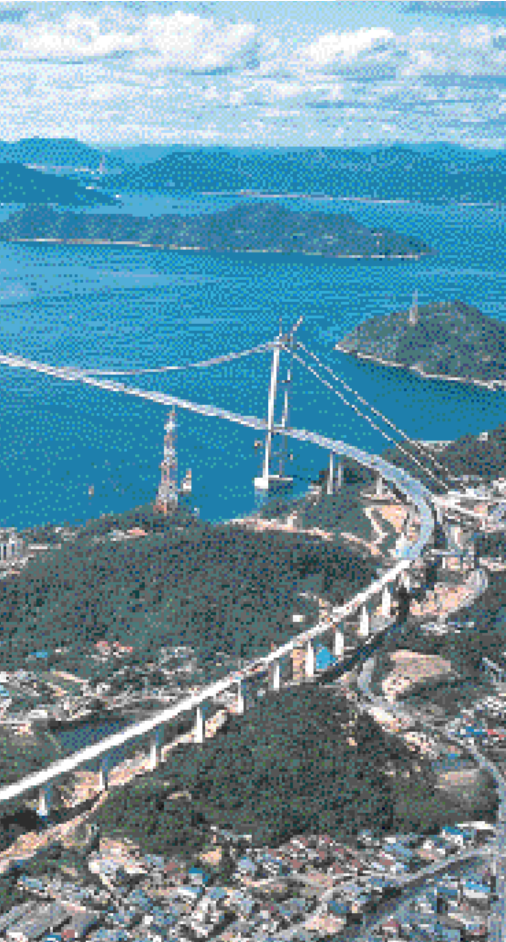
Kurushima Kaiyo Bridge
